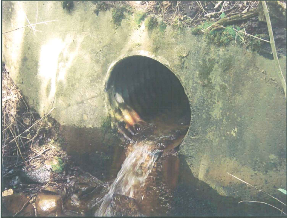
Photograph 3: C-19 (Outlet) – Two foot or Greater Outlet Drop
