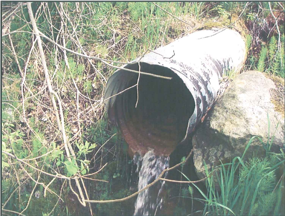
Photograph 4: C-20 (Outlet) – Two foot or Greater Outlet Drop
