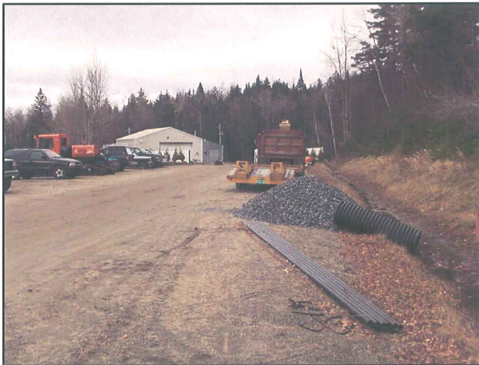
Photograph 16: Subwatershed A32. November 10, 2006
