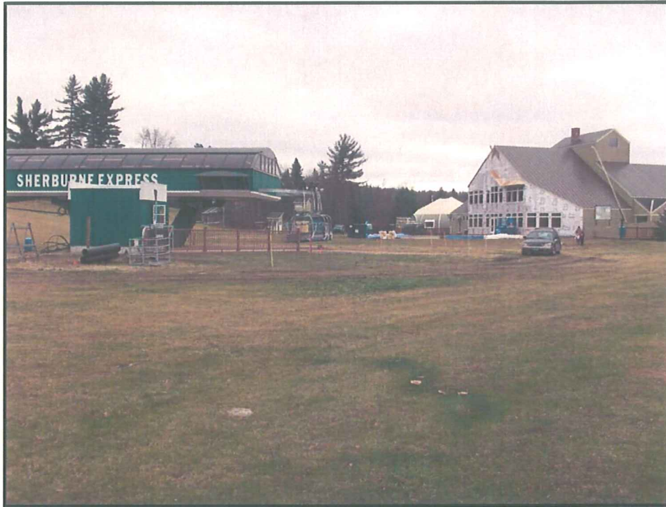
Photograph 15: Subwatershed A13. November 10, 2006
