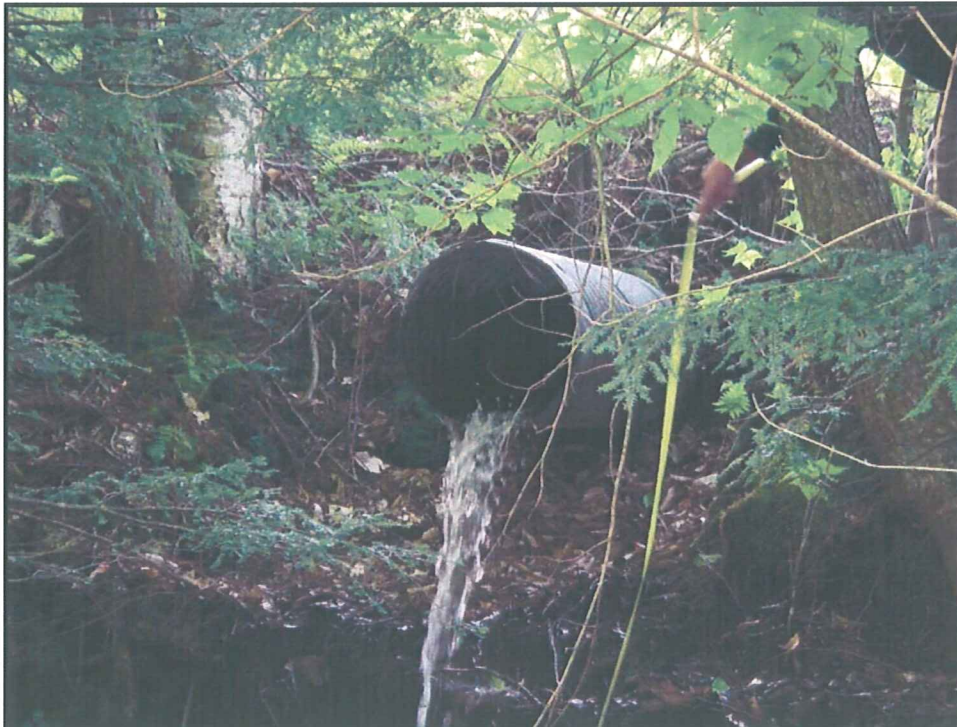
Photograph 2: C-07 (Outlet) – Six foot Outlet Drop
