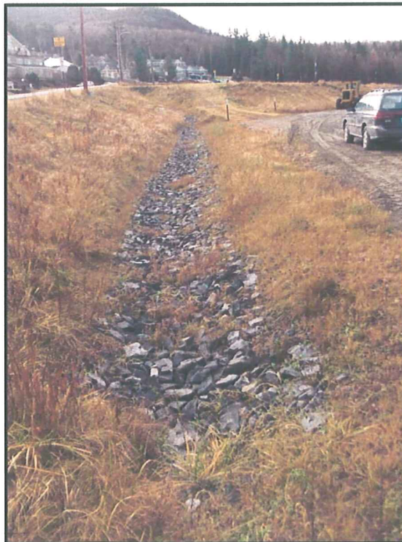
Photograph 18: Subwatershed A42. November 9, 2006
